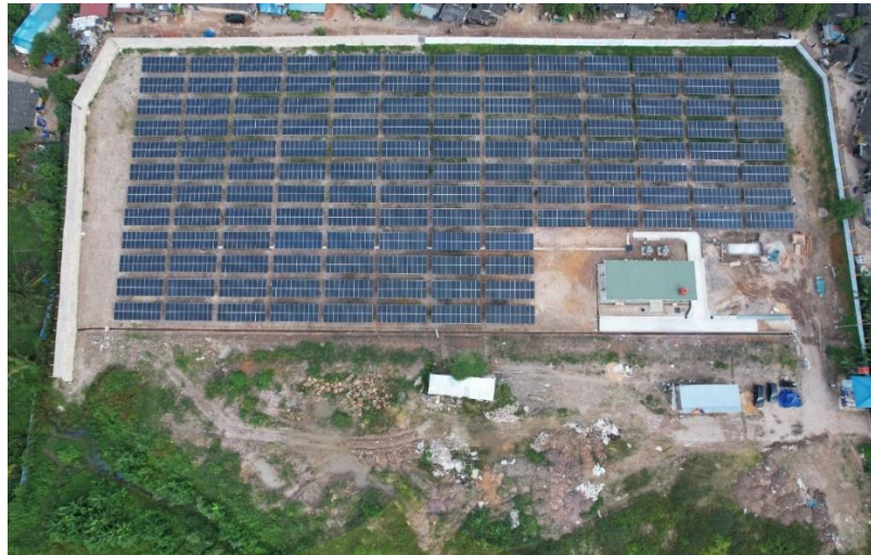
Gambar Metode pemasangan Ground Mounted PLTS 1 MWp Tanjung Uma di Batam
