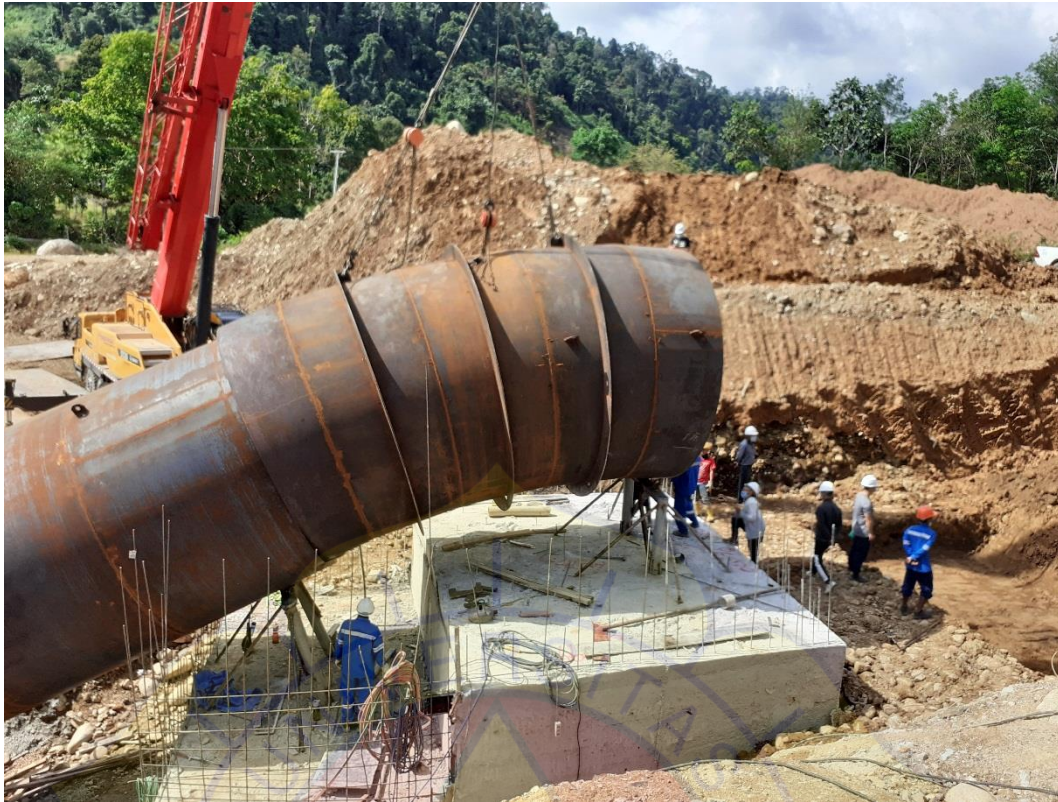
Gambar 6. Pipa Pesat ( Penstock )
