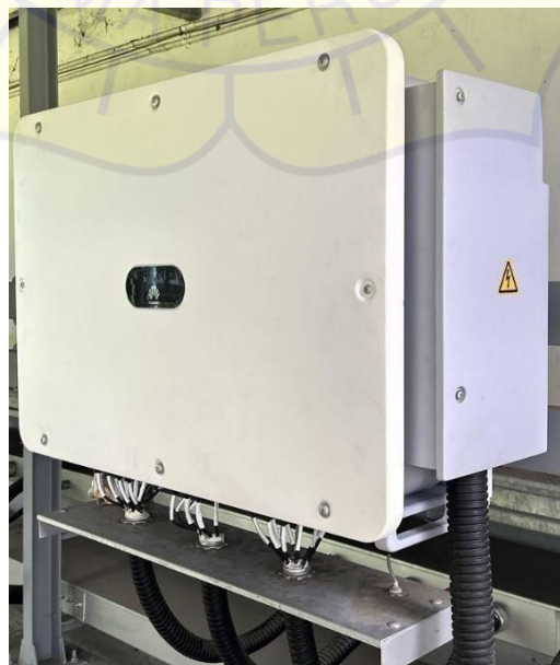
Gambar 2.18 Inverter Huawei SUN2000-100KTL-M2 (Huawei, 2024)
