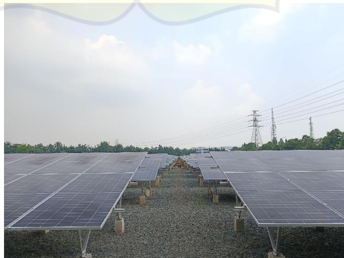
Gambar 2.8 PLTS Ground-Mounted di Kawasan Industri
